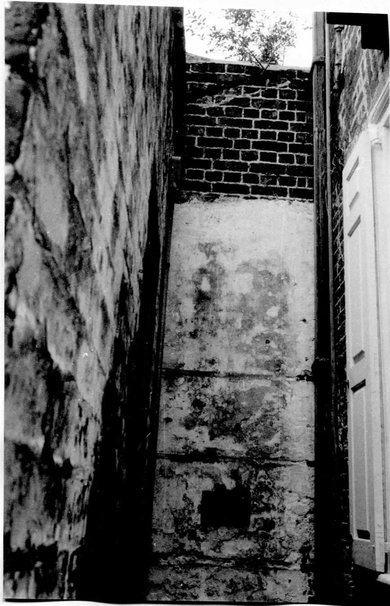
Figure 20. The wall between the back of the Heyward-Washington house and the storage sheds, showing the old roof line at the top and the plaster and ghosting of shelves below.
